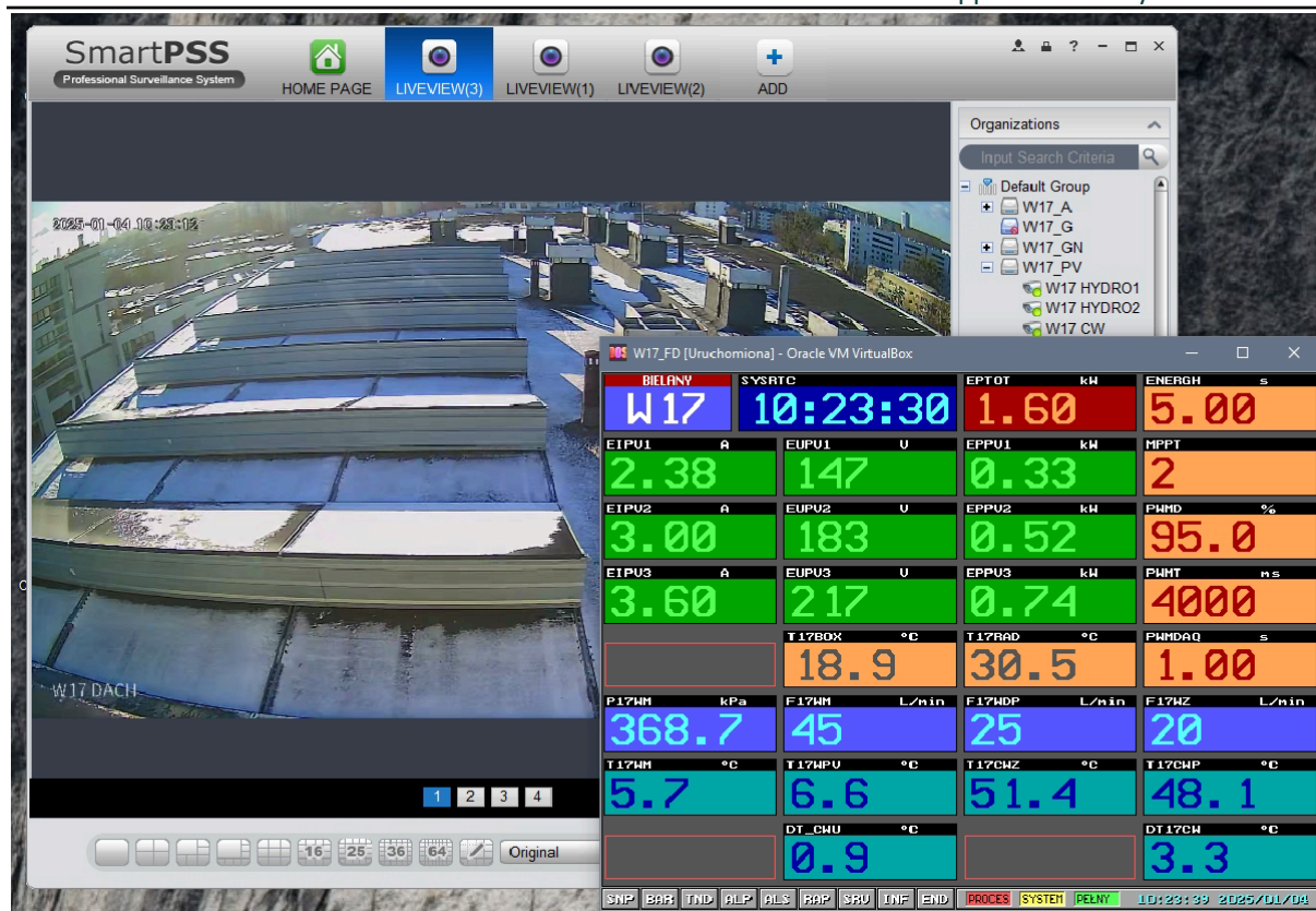
Figure 2. SCADA system monitoring photovoltaics on the roof
